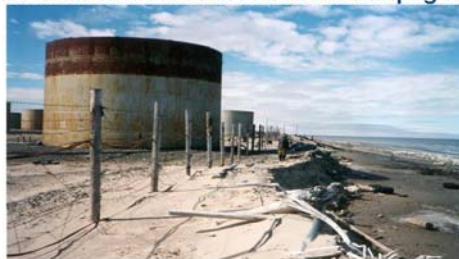
20 years ago these oil tanks were 60 m away from the coast of The Pechora Sea (Ogorogov, 2003)
